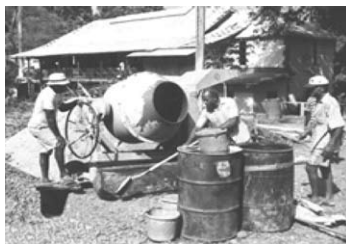
Small-scale Construction and Repair Enterprises
