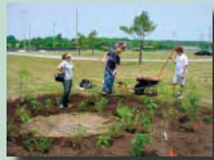
Students install a rain garden on school grounds.
