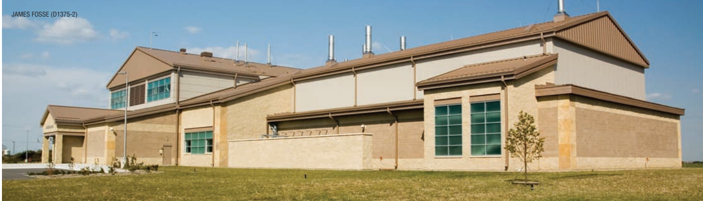
At the National Centers for Animal Health in Ames, Iowa, this state-of-the-art Biosecurity Level 3 animal-containment building is part of the new, larger facility shared by ARS and APHIS.
