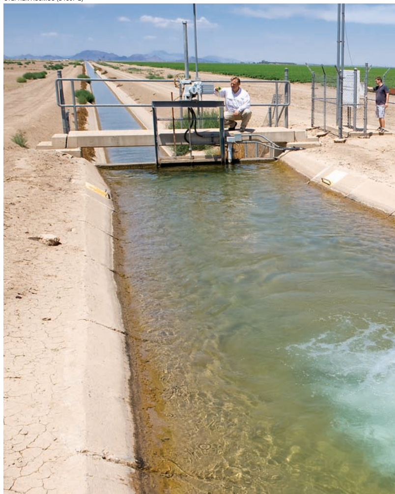
Through a partnership with the Central Arizona Irrigation and Drainage District, ARS electrical engineer Bob Strand (left), ARS hydraulic engineer Bert Clemmens (right), and student Matt Robbins (center) were able to test ARS-developed software on real canals such as this one near Eloy, Arizona.
