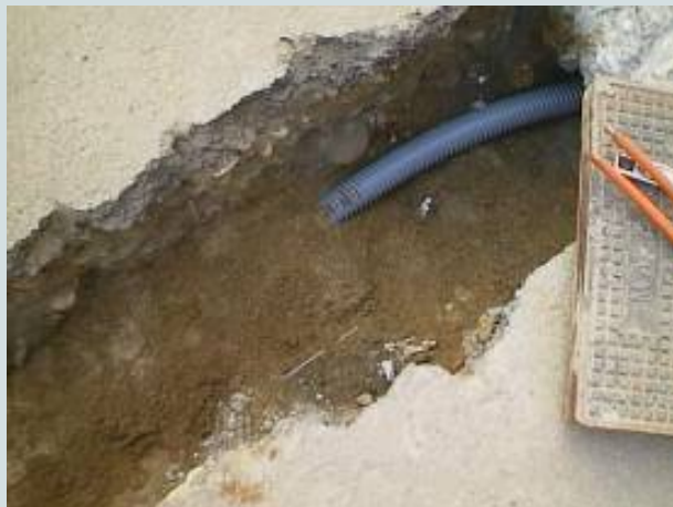
Trench for cables
