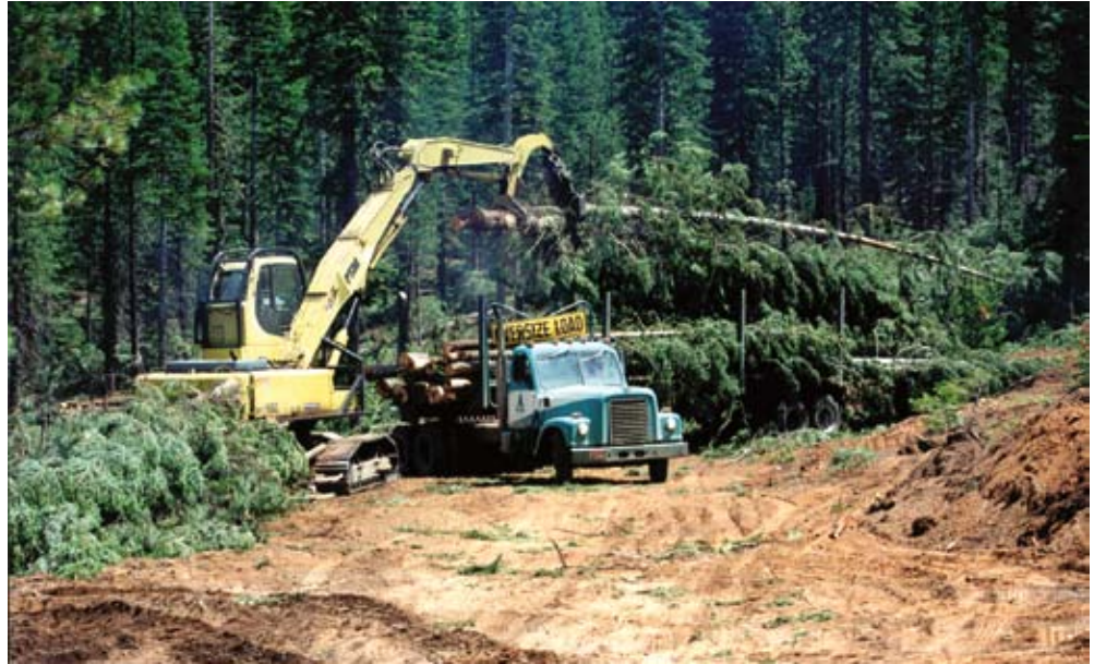
Figure 6—Trees being loaded for transport to the staging area in the Goosenest Adaptive Manage-
