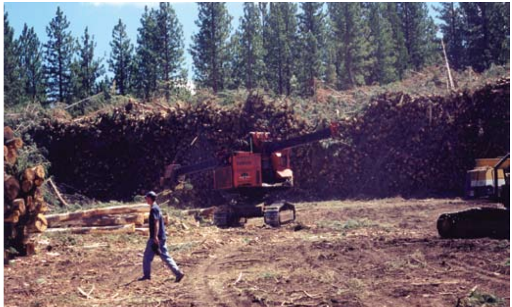
Figure 7—Limbs were removed then, trees were sorted at one of two nearby staging areas.
