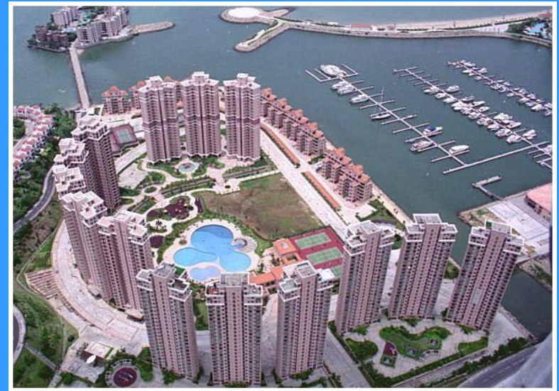
Marina and breakwater development
