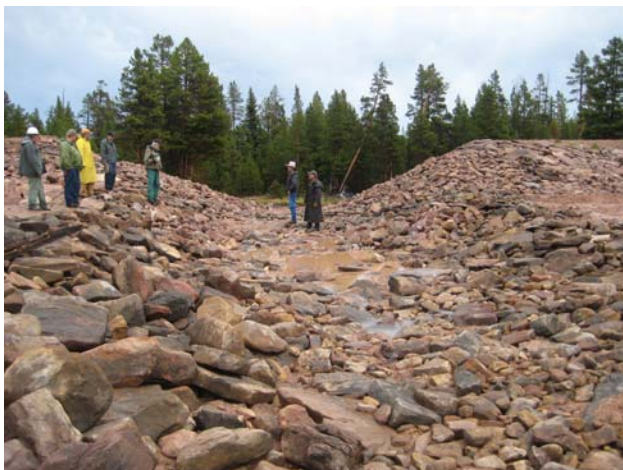
Clements Lake, Dam Breach Final Inspection - (September -2007)
