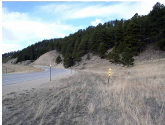
Steep south facing slopes with moderate to heavy fuel loading adjacent to US Highway 16 are a moderate risk for wildland fire.
