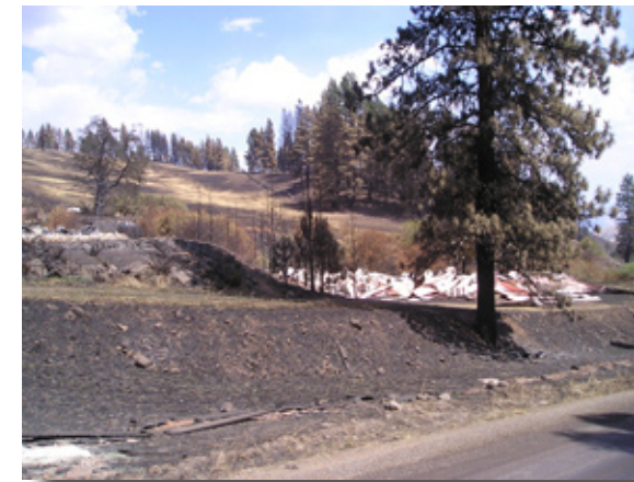
Fire resistant construction materials in conjunction with vegetation treatments may have prevented the loss of this structure.
