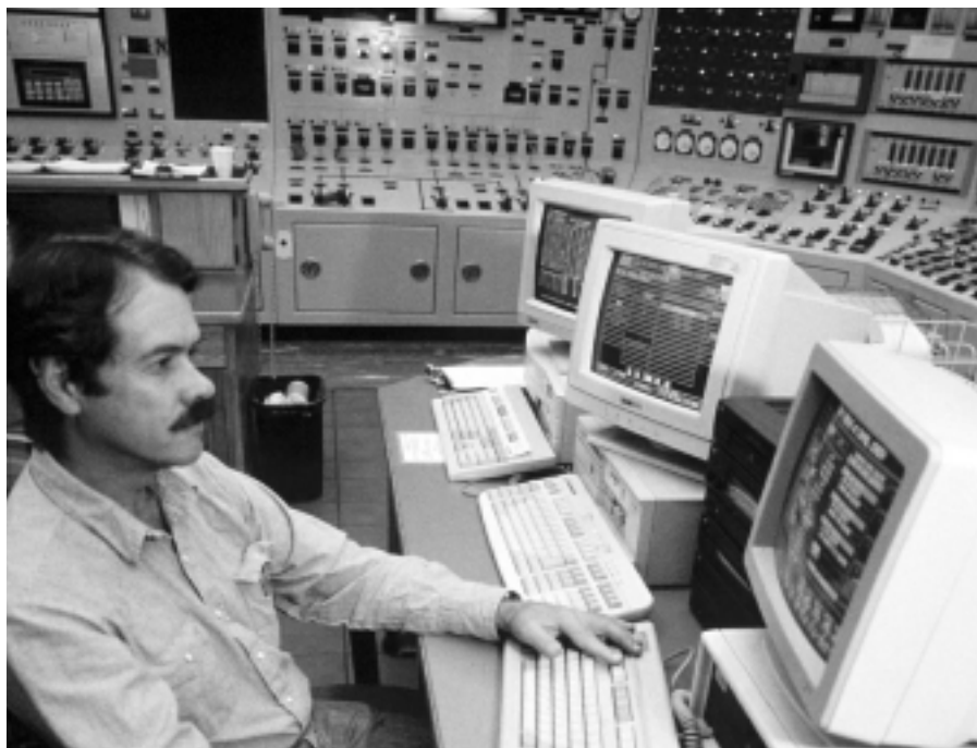
An employee of an electric power cooperative monitors power distribution to customers.
