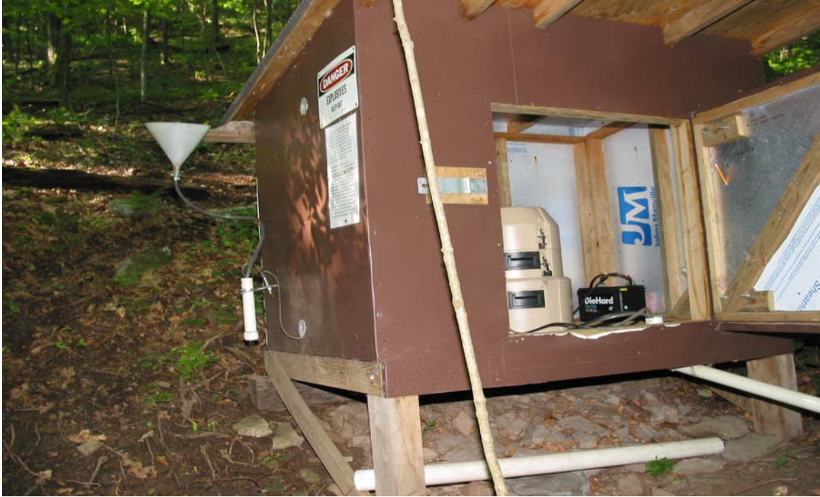
Figure 2. A constructed monitoring station used to collect water samples and record streamflow velocity.
