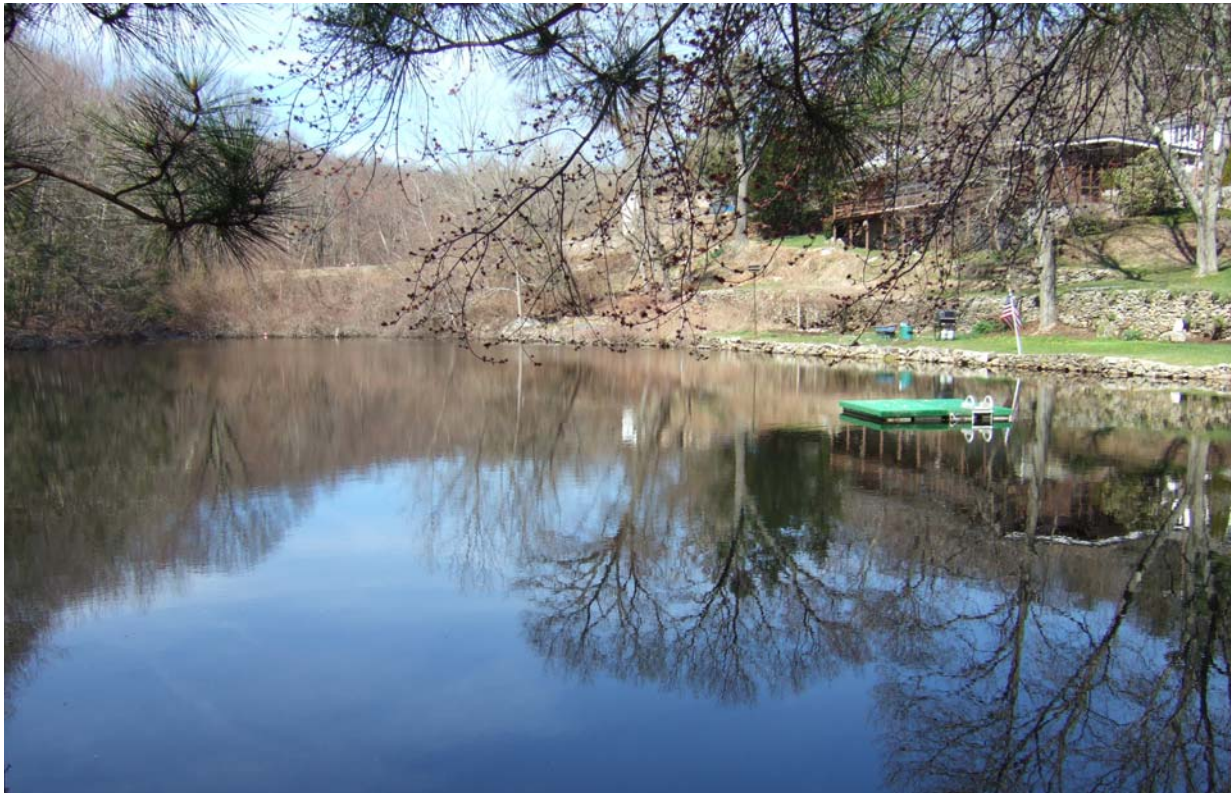
Figure 4. 5 Impoundment of the Hughesdale Lower Pond Dam
