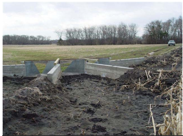
Figure 4. Rear view of flumes showing wing walls and burms.
