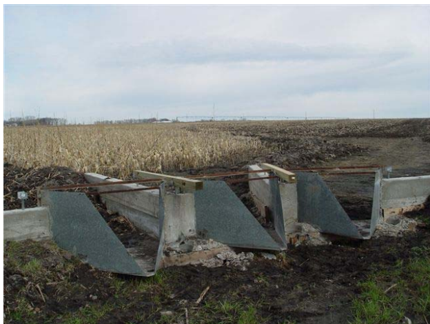
Figure 3. Front view of watershed flumes at the runoff discharge site.
