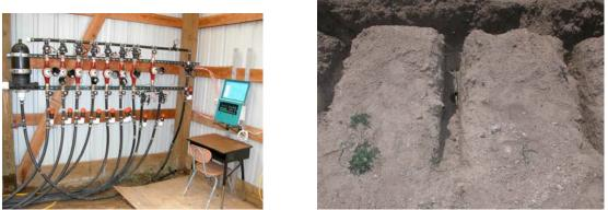
Figure 2 – Computer and valve controls for the SDI research site and open trenches for SDI lines.
