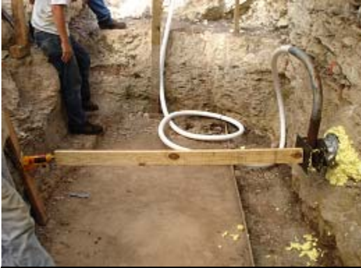
Injector apparatus in the trench
