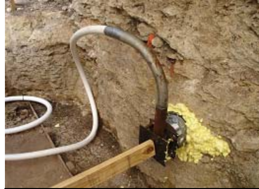
Injector apparatus in the trench
