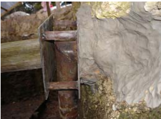
Seal and injection head
