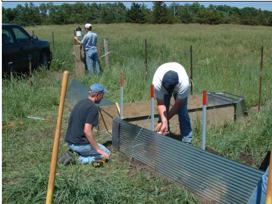
Figure 2 - Installation of sampling equipment on tile/grass waterway.
