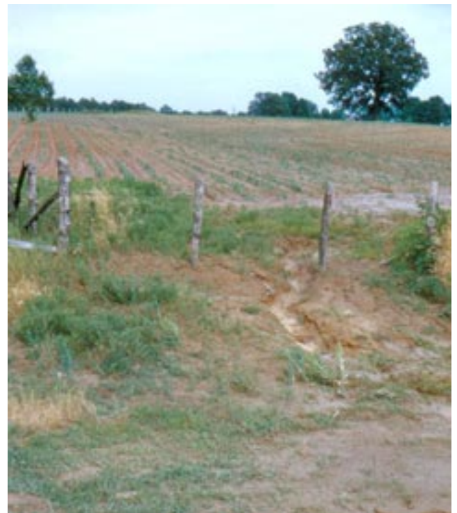
Figure 2.—Runoff and erosion after heavy rains can create serious sedimentation problems on local roads.
