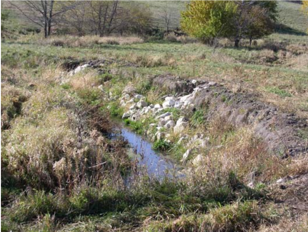
Figure 11.—Streambank stabilization practices help to control erosion along stream beds.
