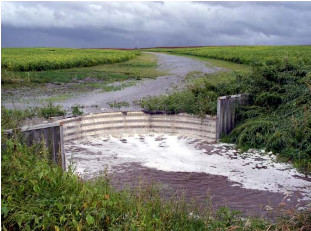
Figure 12. —Grassed waterways and drop structures help to convey runoff from areas of cropland at a nonerosive rate.
