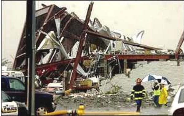
Fun Zone Skating Rink and day care center destroyed by an F2 tornado in Montgomery, Ala. (Photo: Courtesy WSFA-TV)
