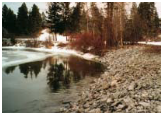
Rock riprap and soil were used to stabilize the Stillwater River near Kalispell.
