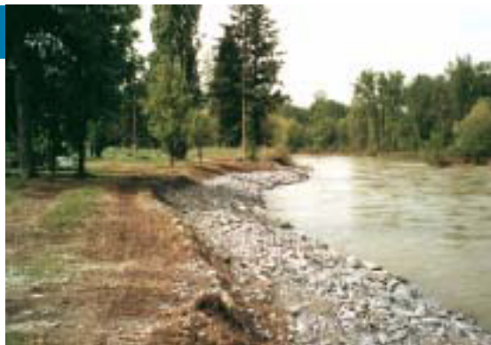
Approximately 500 feet of rock riprap was used to control erosion on the Stillwater River near Kalispell.
