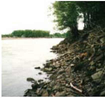
Bendway wiers along the Yellowstone River will protect property from future flooding.
