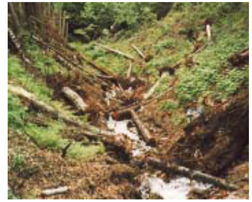
EWP funds were used to repair an eroded drainage area into the Thompson Falls' drinking water collection site that was allowing high sediment loads to enter the water supply.
