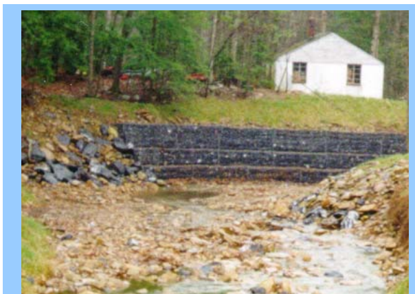
Fig. 2.3-5. Gabions Installed at Rocky Run, VA
