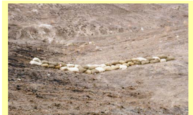
Fig. 2.3-19 Temporary Grade Stabilization Structure, 8th Street Burn, Boise Hills, ID
