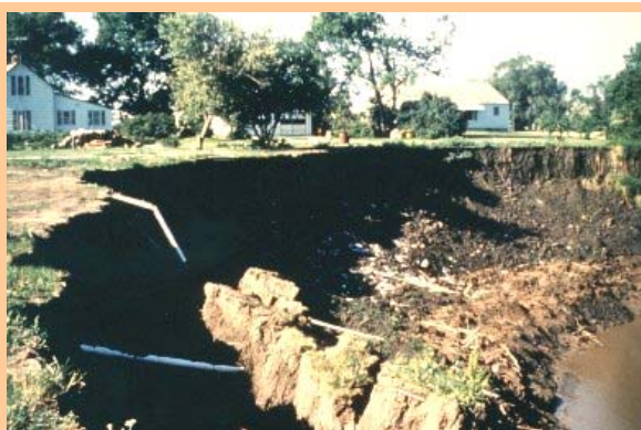
Fig. 2.3-4 Property Threatened by a Failed Streambank
