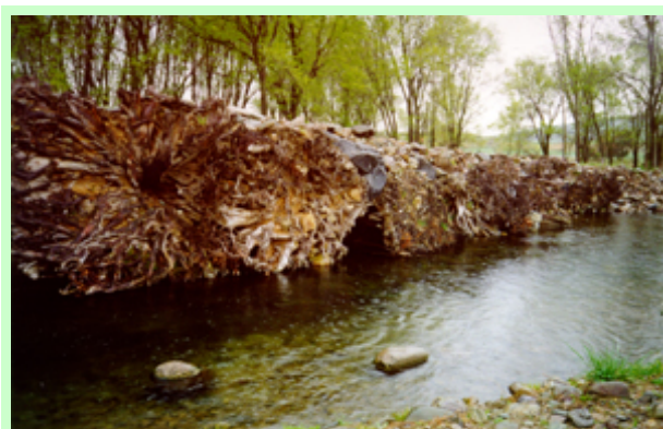
Fig. 2.3-7 Rootwads Installed at Rose River, VA
