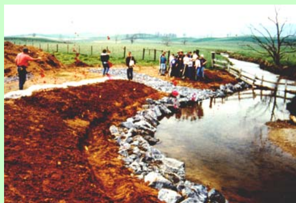
Fig. 2.3-10 Bank Vegetation Site, Back Creek, Augusta County, VA (with riprap toe section)
