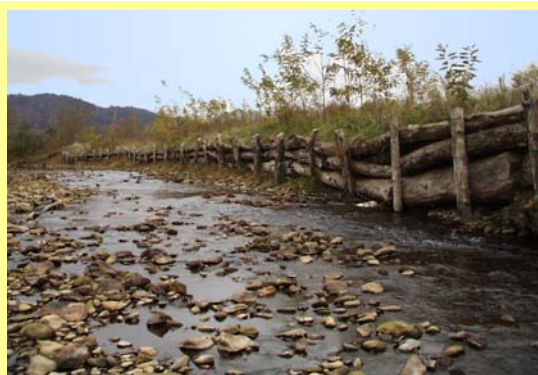
Fig. 2.3-8 Timber Cribbing Structure, Cherokee County, NC
