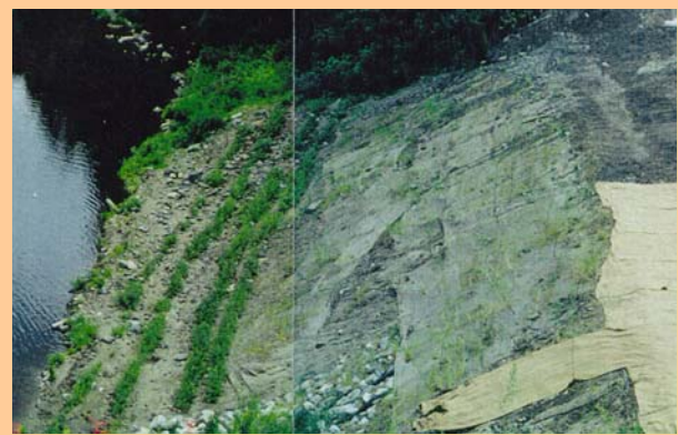
Fig. 2.3-9 Composite photo, live plantings in rock base (left) and soil bioengineering using geotextiles, Glen Arbor, Santa Cruz Co., CA
