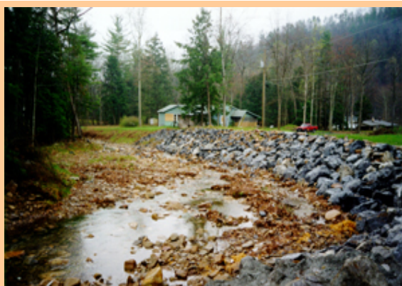
Fig. 2.3-6 Riprap Installed at Rocky Run, VA
