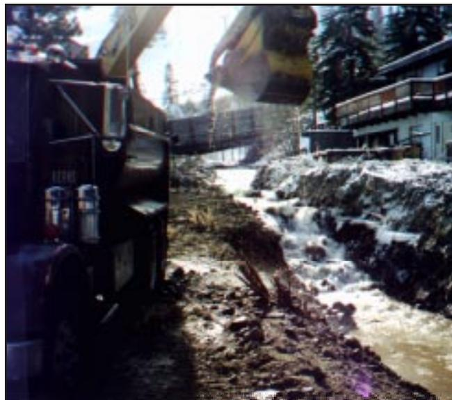
*Shown above, sediment removal and rechannelization work along the South Fork Squaw Creek. Note the original elevation of debris on the right side of the creek. Shown below, the creek after emergency work to divert water flow back to the existing channel. The debris piled up to the top of the deck rail on the left, about 8 feet above the top bank of the creek.*
