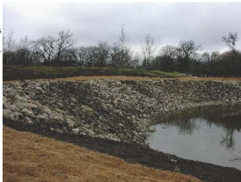
October 2003 Bank stabilization complete in Hallock
