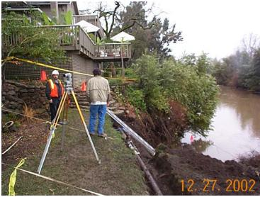
Heavy rains and flood stage waters on the Napa River led to severe streambank erosion and land subsidence in the vicinity of the main resort building at the Milliken Creek Inn. NRCS determined that the building was imminently threatened by further rainfall and high river stage. EWP work commenced within 24 hrs. of the declaration, on December 19, and was completed January 10.
