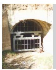
Local residents were concerned about this culvert in the Malibu Creek watershed in Calabasas (shown left). Debris washed down the channel during heavy rains would pile against the grating and quickly clog the opening. To prevent this, EWP crews cleared brush and debris from about 1,500 feet along the channel (top right). The debris was then chopped up (bottom right) and deposited on the channel banks.
