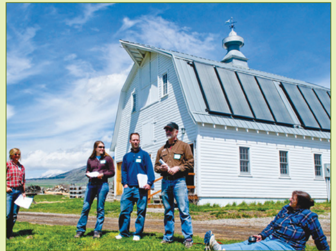
Solar hot water panels line the roof of the barn at 13 Mile Lamb and Wool company in Belgrade.
