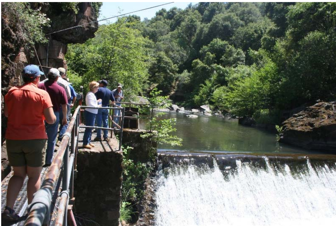
Wildcat Dam to be removed in project to restore fish passage for Chinook salmon and steelhead on the North Fork of Battle Creek
