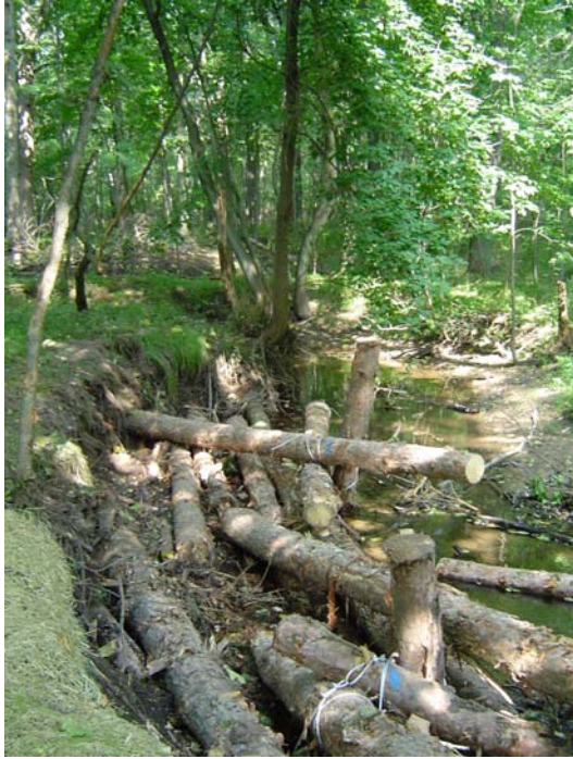
Lancaster Brook Stream Restoration
