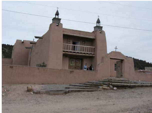
Authorized in 2006, the Northern Rio Grande NHA works to preserve and interpret historic structures in the region, including traditional Adobe buildings such as the San Jose de Gracia NHL in Trampas, New Mexico.
