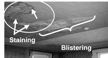
Water stains and examples of paint blistering and wall paper (above and below), peeling
