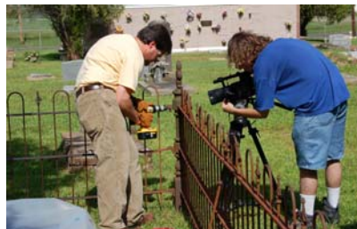
Jason Church, NCPTT materials conservator, demonstrates the proper method to remove a broken bolt during filming of the Basics for Iron Fence Care video. (Stace Miller)
