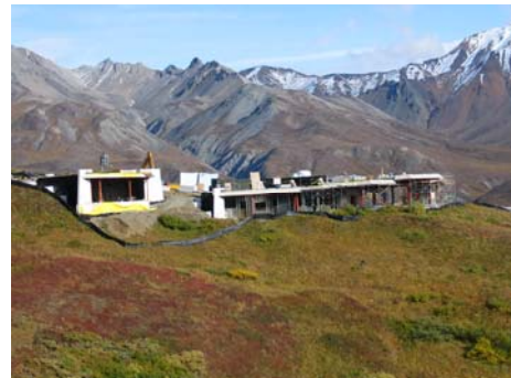
Construction on the Eielson Visitor Center, Denali NP & Pres
