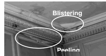
Water stains and examples of paint blistering and wall paper (above and below), peeling
