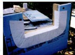
WINDOW/DOOR PAN FLASHING
