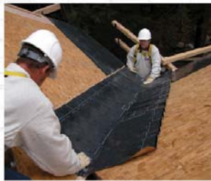
BITUMINOUS MEMBRANE AT VALLEYS
