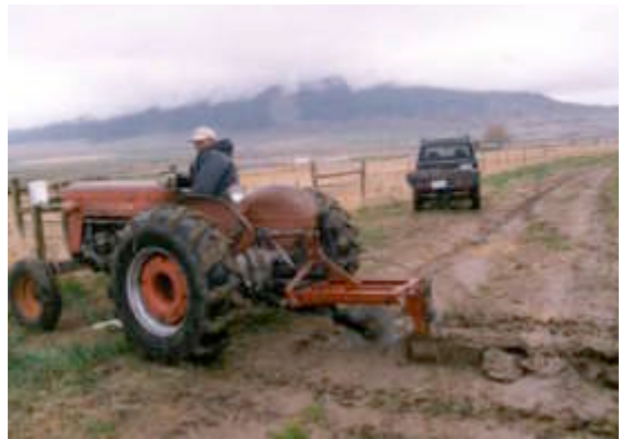
Home-made cable-laying implement. (NCAT photo)
