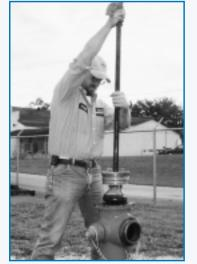
6. Use the manufacturer's seat wrench to unscrew the seat ring.
