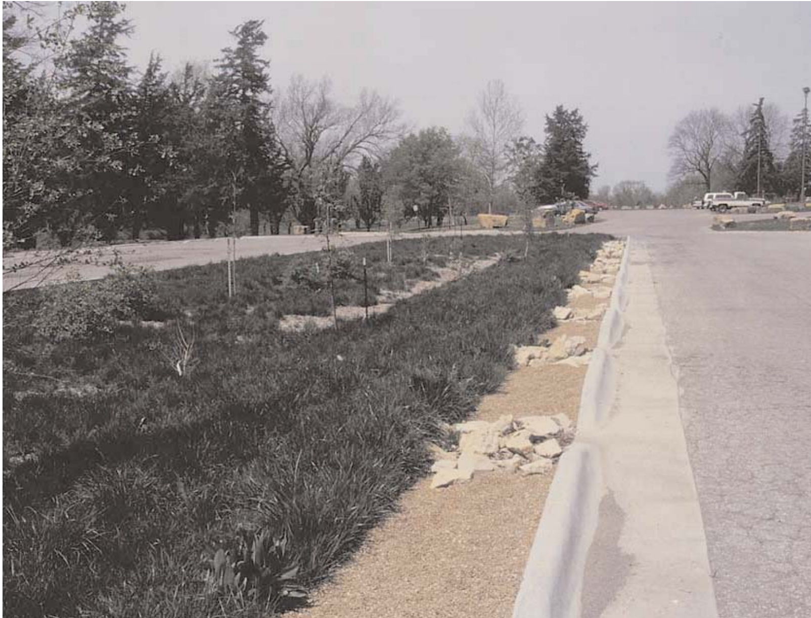
This newly constructed bioswale in the Hillcrest Community Center's parking lot helps to reduce storm-water runoff volume and improve water quality.
