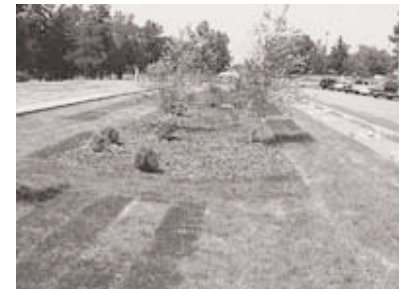
This newly constructed bioswale in the Hillcrest Community Center's parking lot helps to reduce storm-water runoff volume and improve water quality.
