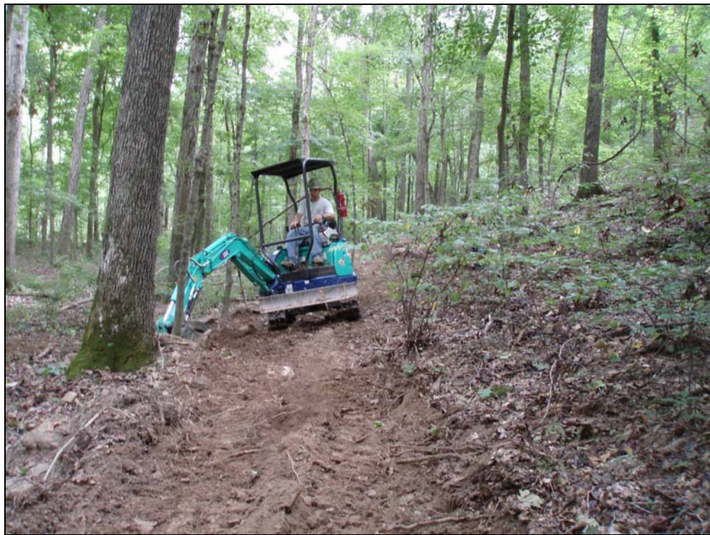
Figure 3. Mini-excavator being used to install drainage dips on re-route.
