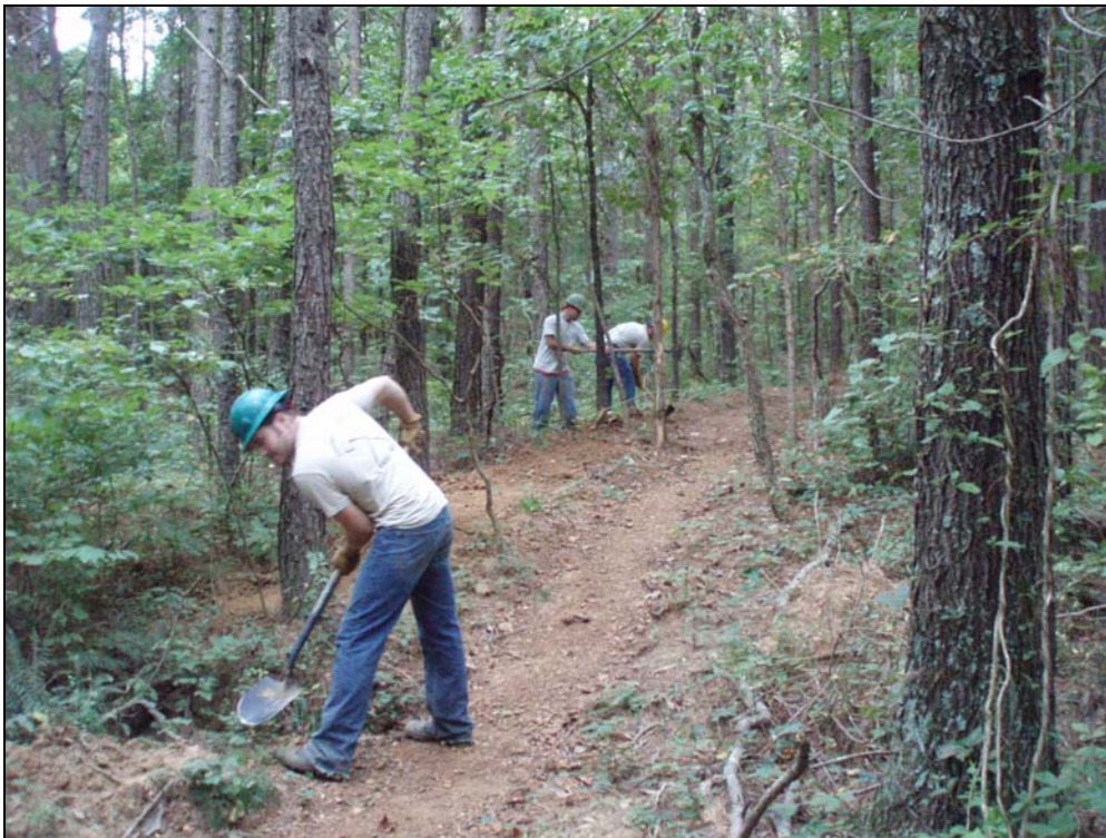
Figure 4. Trail crew member clearing an outflow ditch along the trail.
