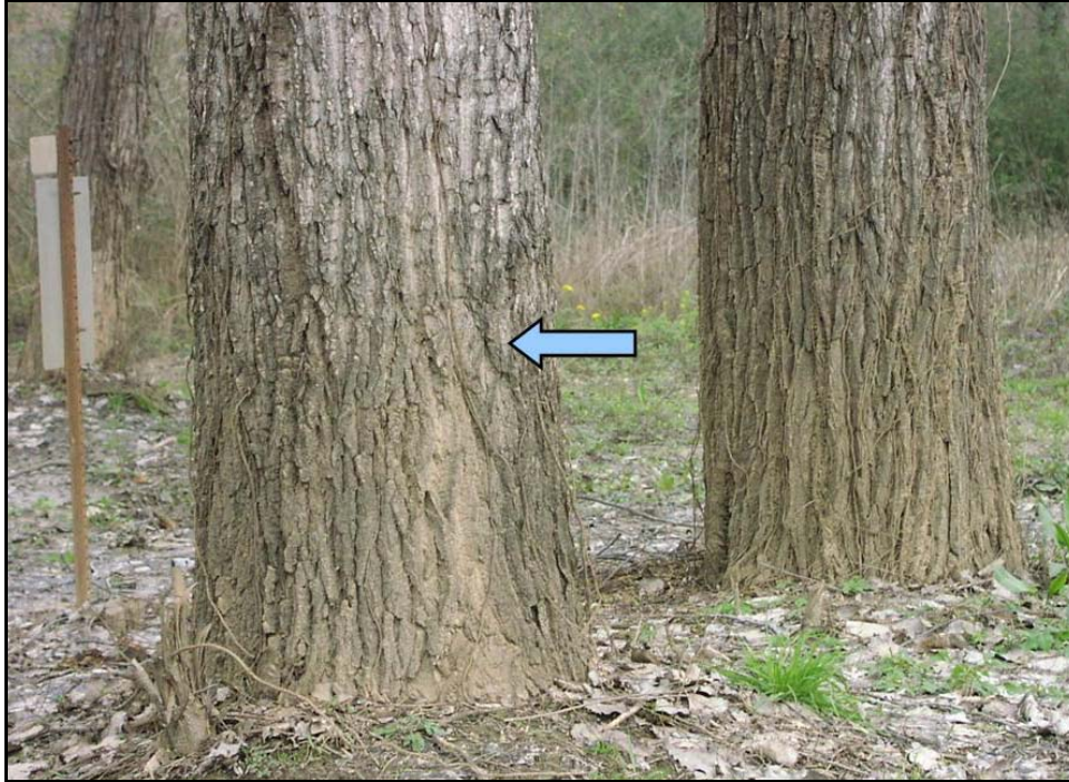
Figure 27. Silt deposit left after a recent high-water event forms a tan coating on these tree trunks (upper edge indicated by the arrow).
