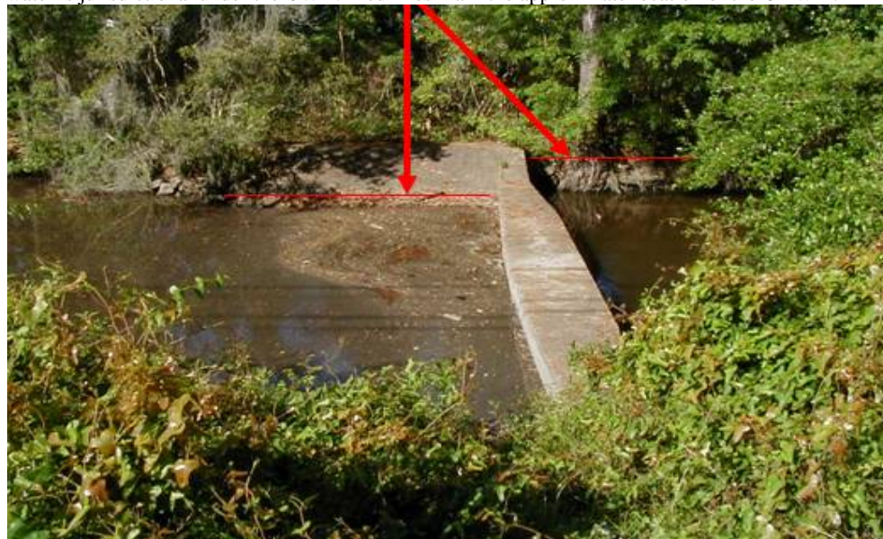
Photo 42. Impoundment on an RPW, South Atlantic Division. Water flows into a TNW; water is jurisdictional under the CWA. Red lines mark the approximate location of the OHWM.
