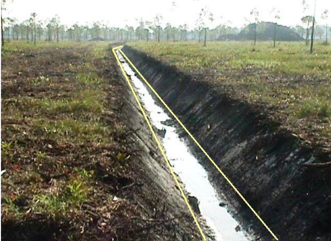
Photo 53. Drainage ditch, an RPW, South Atlantic Division. Ditch excavated in wetlands; ditch is subject to jurisdiction under CWA. Yellow lines mark approximate location of OHWM.
