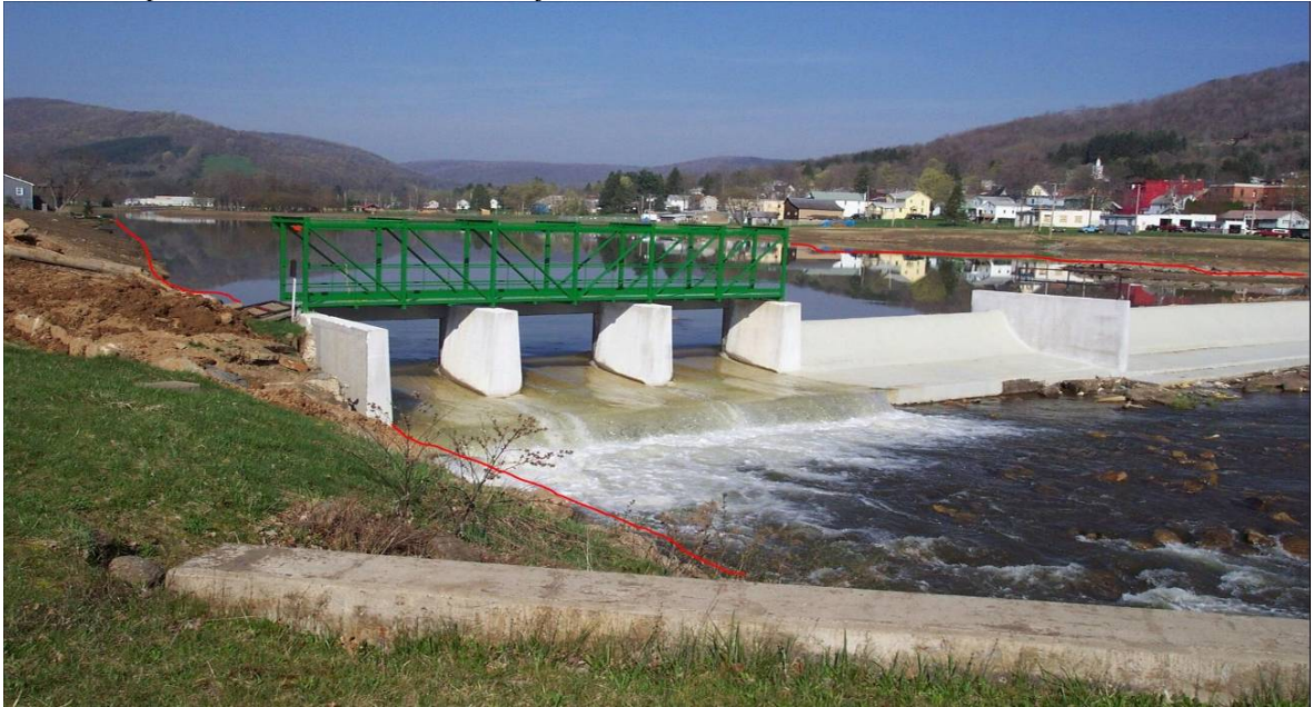
Photo 41. Impoundment on a TNW, PA; water is jurisdictional under the CWA.
