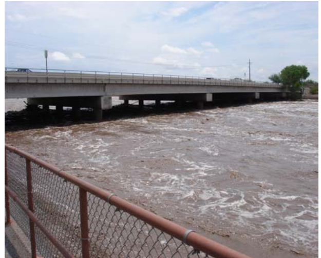
Photo 25. Rillito River (ephemeral tributary), AZ. Flow is following a 3" rainfall event.
