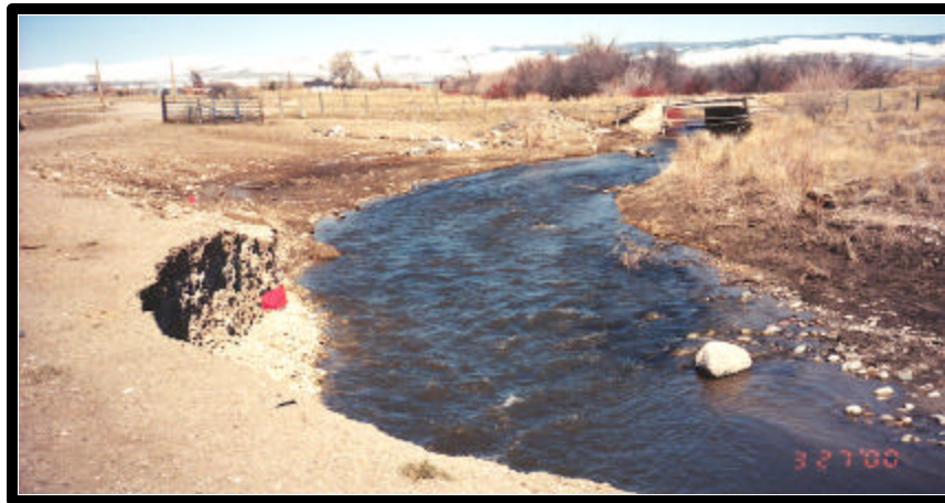
Figure 1: Eroding bank on the Jack Webster Ranch, lower end of Medicine Lodge Creek about 15 miles West of Dubois, ID in March, 2000.
