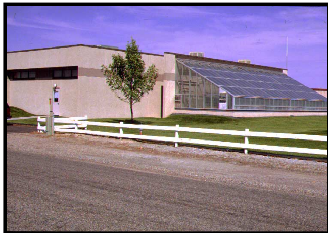
Aberdeen Plant Materials Center office and greenhouse
