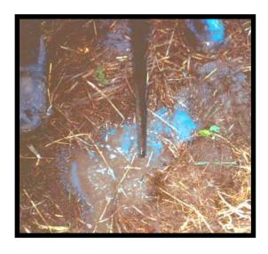
After turning on the ball valve and the water starts jetting out of the nozzle, the waterjet will slowly start sinking into the ground. If a hard layer is encountered, the waterjet will stop. If the user leaves the waterjet in place and let the water work on the layer, eventually it will go through it. We have demonstrated this with several demonstration projects from a site with a 6 in hard calcic layer to a site with a 2 ft thick layer of decomposed granite. If medium sized rocks (with
