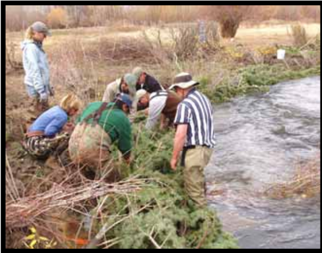
Workshop participants install brush revetment on the Lemhi River
