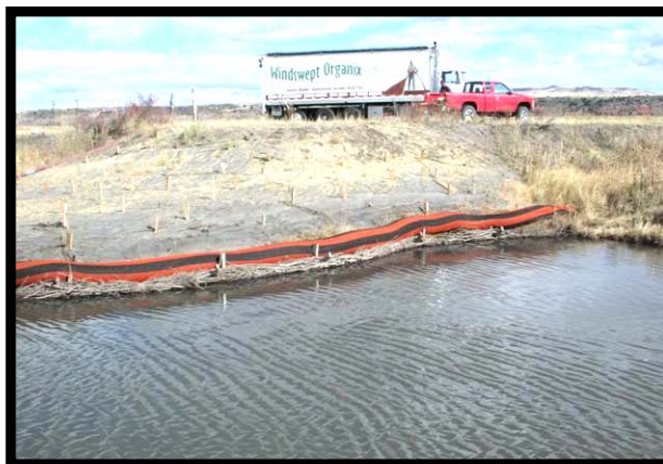
Testing a new organic soil-filled sack for a fascine on the Little Colorado River, AZ
