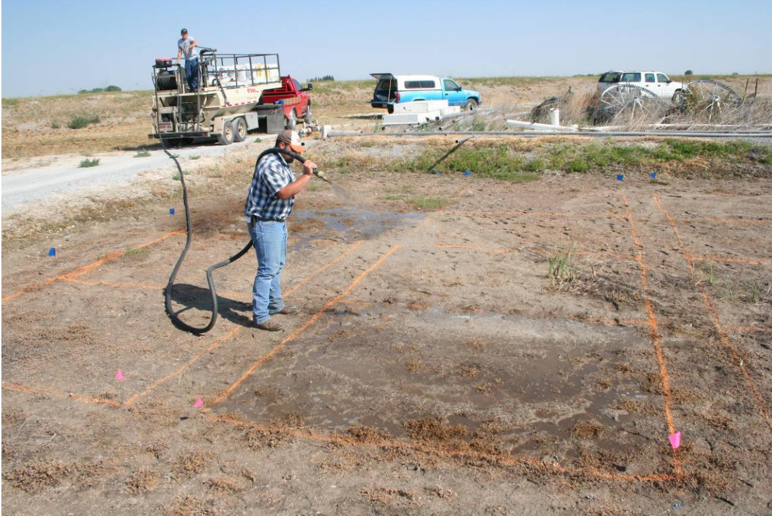
Hydroseed application of Fertil Fibers treatment.
