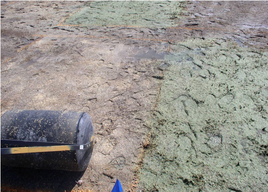
Rice hulls and seed pressed into soil with roller.
