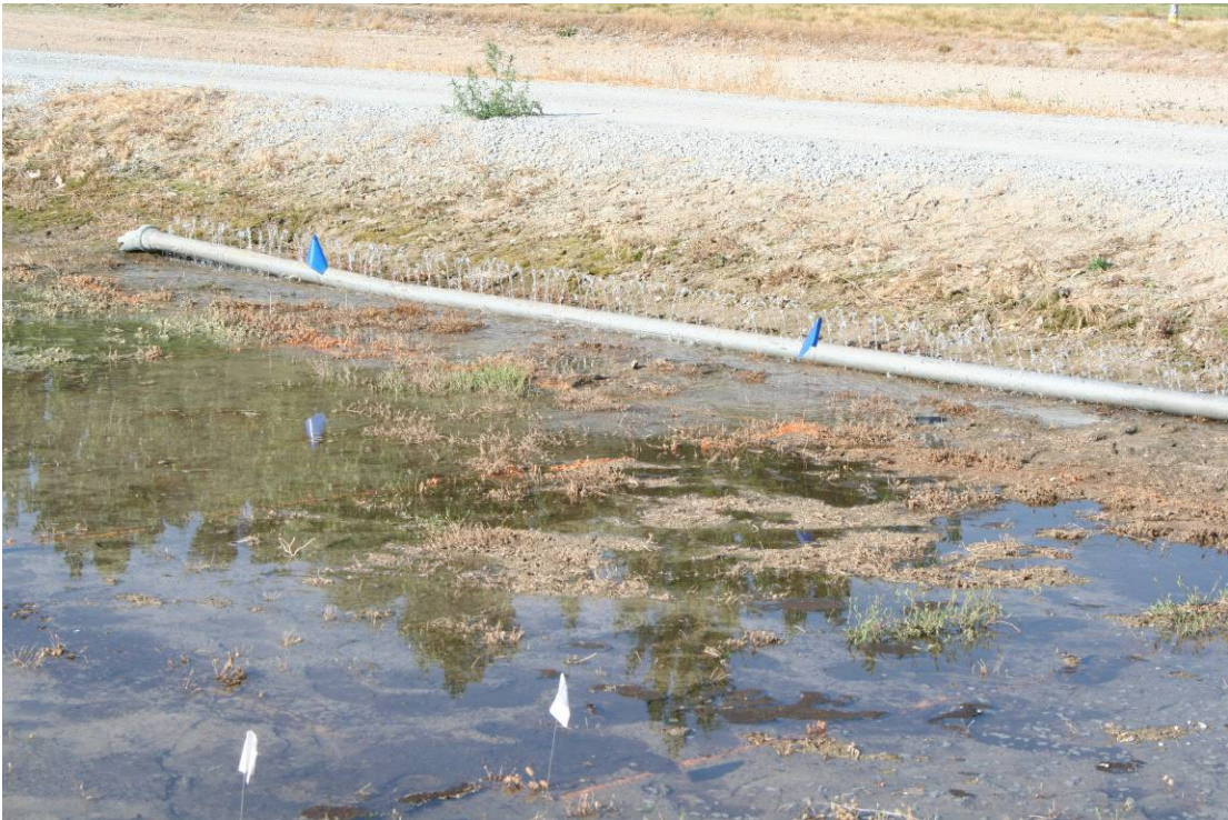
Perforated irrigation pipe watering the pond.
