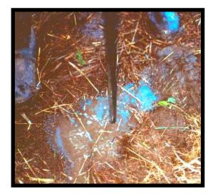
After turning on the ball valve and the water starts jetting out of the nozzle, the waterjet will slowly start sinking into the ground. If a hard layer is encountered, the waterjet will stop. If the user leaves the waterjet in place and let the water work on the layer, eventually it will go through it. We have demonstrated this with several demonstration projects from a site with a 6 in hard calcic layer to a site with a 2 ft thick layer of decomposed granite. If medium sized rocks (with
