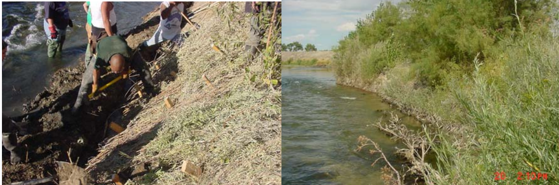
Figure 4: Brush Mattress under construction and after 2 years.
