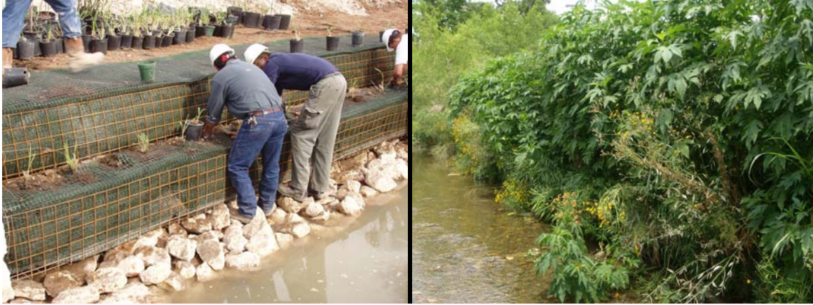
Figure 3: Vegetated wire face MSE wall. Under construction and after 2 years.
