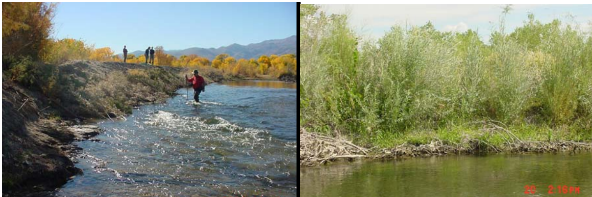
Figure 5: Vertical bundles and brush revetment. Under construction and after 3 years.
