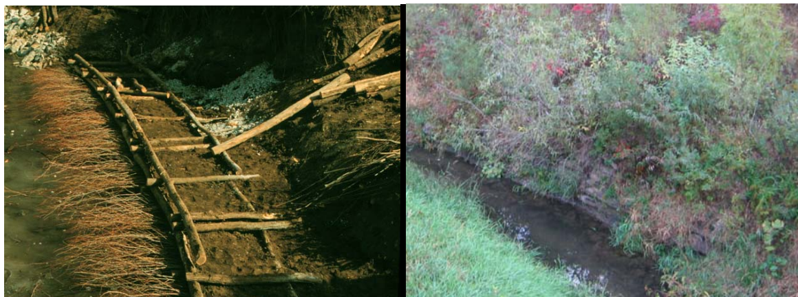
Figure 2: Log Crib. Under construction and after 10 years
