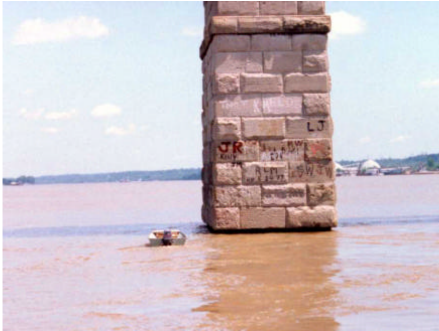
Figure 42. Remote-control boat being tested near a pier.
