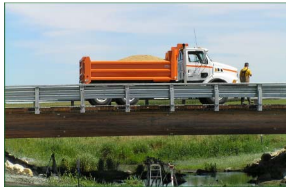
Glued-laminated bridge reinforced with FRP laminations.
