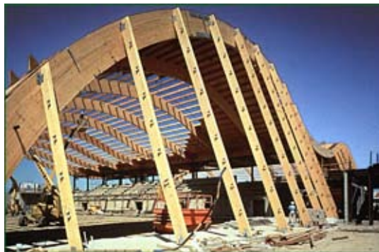
Use of curved glulam beams at the Disneyland Ice Arena, Anaheim, California.
