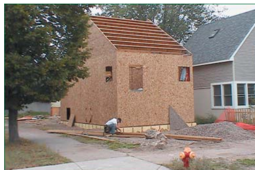
Demonstration House 2 with SEP walls completed and waiting for the roof deck. To the right is the completed and occupied Demonstration House 1.
