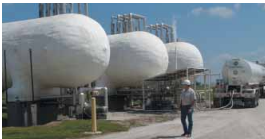
Clockwise from upper left: ethanol and corn samples are tested in the lab at the NEMO plant; MidMo (next two photos) plans to double production capacity, to 100 million gallons; NEMO Plant Manager Steven Burnett checks on the CO 2 plant, which supplies a brewery and other beverage customers; Ryland Utlaut, center, in the receiving room at MidMo. USDA photos by Dan Campbell
