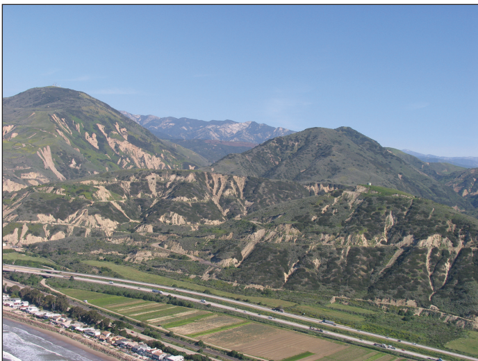
Landslide scars above US 101 west of Ventura. Photograph by Jonathan Godt, March 2005.
