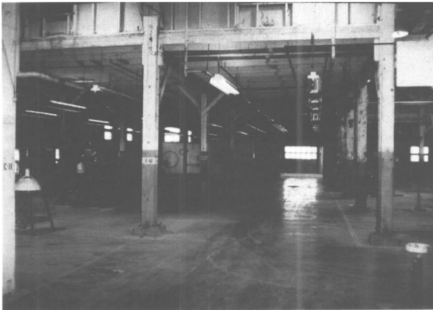
Figure 1. —The 8- by 8-columns supporting the mezzanine floor of building 503.
